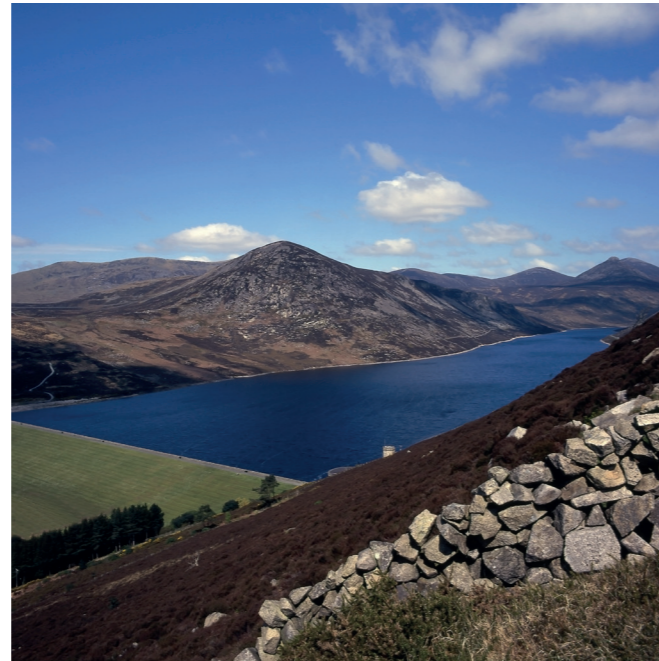
Normal water levels at the Silent Valley reservoir, County Down Image courtesy of Northern Ireland Water
