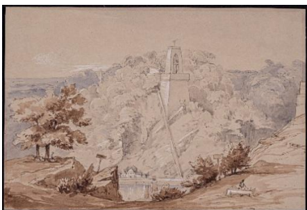
View of the bridge
