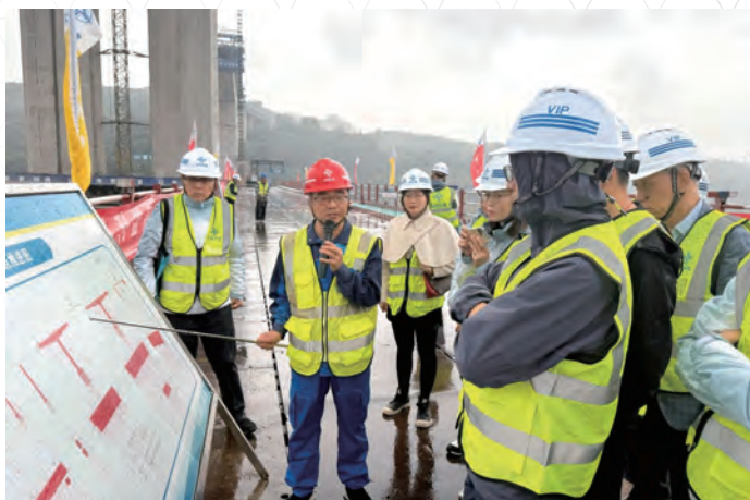
Site visit to Baoshan Jialing River Bridge project
