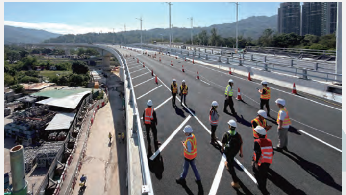
Site visit to the horizontal vehicular bridge rotation operations
