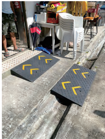
Ramps installed to improve accessibility for wheelchair users
