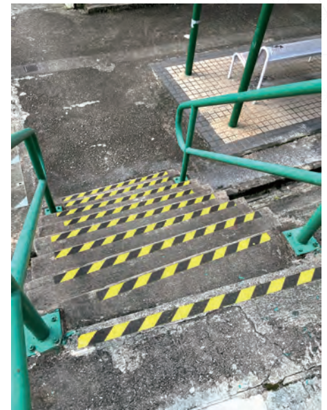
Anti-slips installed to improve safety of villagers
