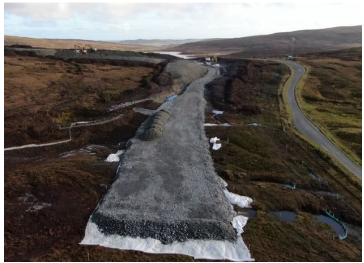
Viking Wind Farm Construction of New Sandwater Road
