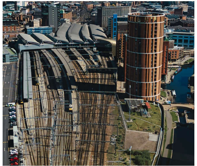
The Transpennine Route Upgrade, one of Julie's major projects
